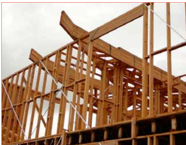
Trusses are design specific for each house so it is uncommon for trusses to be stolen from site. They are often delivered to site and stacked on top of the wall frames.
