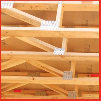
The high performance cost effective system using steel or timber webs
