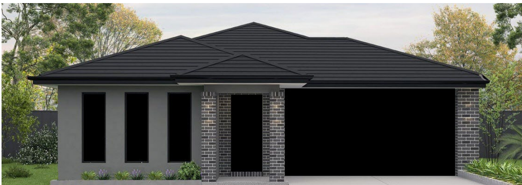
Fig 1 - Typical examples of front elevations with short walls where a PMB would be best suited.
