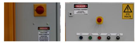
On the front door of the electrical control cabinet is an illuminated push button that, when the FNR press is first turned ON, it illuminates to show that the emergency system requires resetting. When the emergency system has been activated and then cleared, the Blue colour RESET button will flash and will require pressing to reset.
