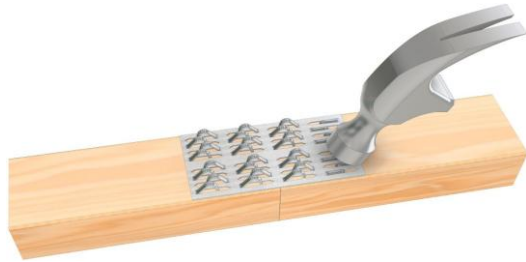
Hammer Parallel to Nails
