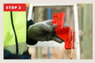
Take an Internal Wall Screw and place it in the slot on the guide. Using the guide will ensure the screw is positioned in the correct location.
