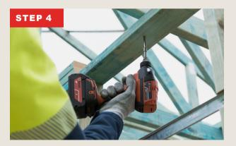
Remove the guide once the netsetter meets the guide and drive the screw home.
