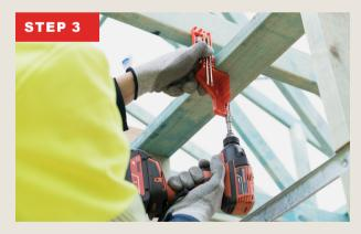
Place the guide to the underside of the wall frame and move the guide until it's resting up against the roof truss. Drive the screw until the nutsetter meets the guide.
