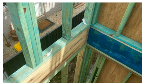
175mm for double top plates to beam connection
