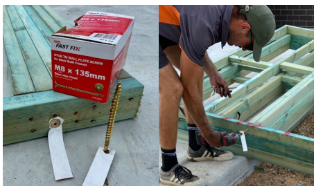
135mm for single bottom plate to stud connection
