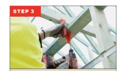
Place the guide to the underside of the wall frame and move the guide until it's resting up against the roof truss. Drive the screw until the nutsetter meets the guide.
