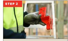
Take an IWS and place it within the hloding slot on the guide. Using the guide will ensure the screw is positioned in the correct location.
