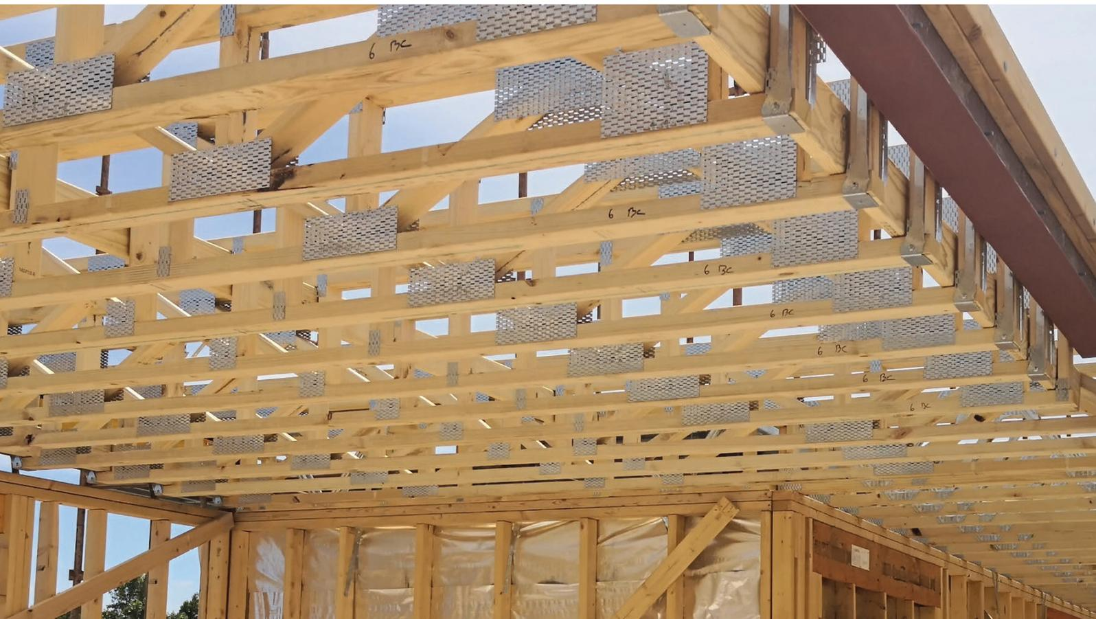
Another key benefit of Pryda's truss system is open web configuration that eliminates potentially damaging building practices, such as cutting out sections for services or drilling large holes. Large rectangular ducts up to 500mm wide fit within the standard design.
